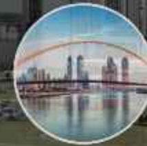
Dubai Water Canal
